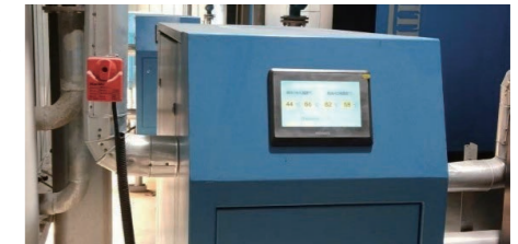
Waste Heat Recovery Transformation of Air Compressor
